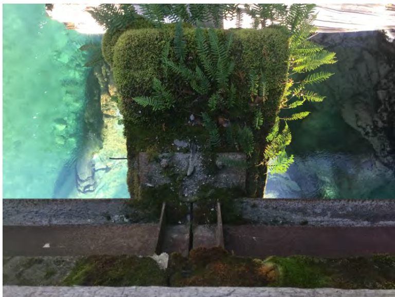
Upstream left pier bearing
