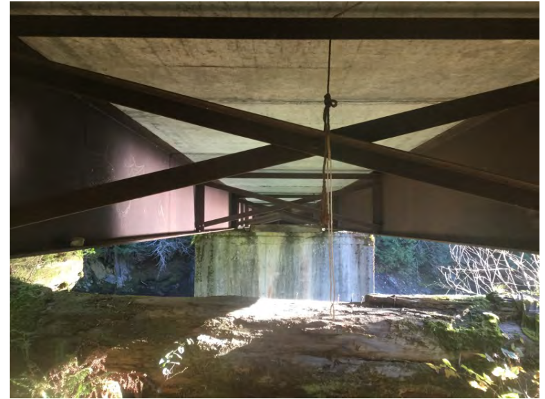
Right span superstructure
