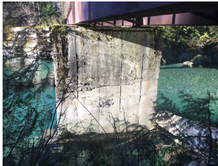
Left face of left Pier
