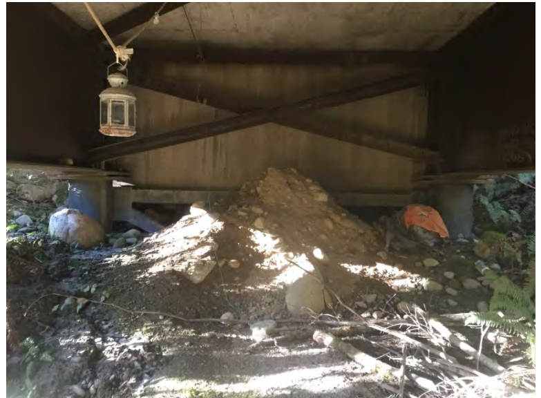
Right Bank Abutment when facing downstream
