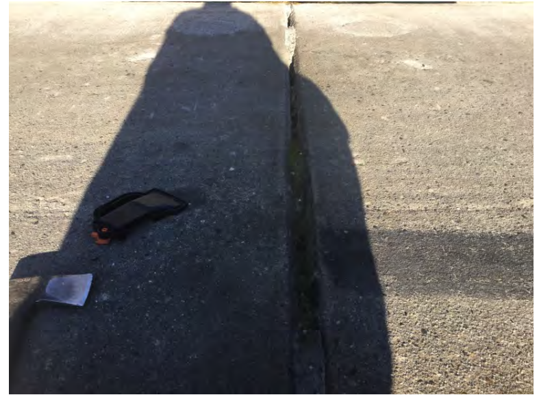
Right Pier deck joint
