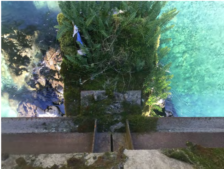
Upstream right pier bearings
