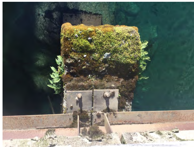
Downstream left pier bearings
