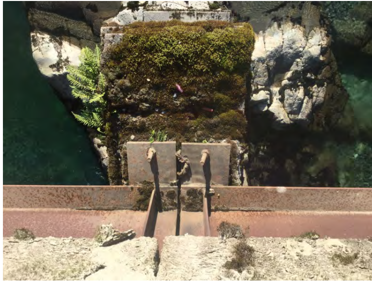
Downstream right pier bearings
