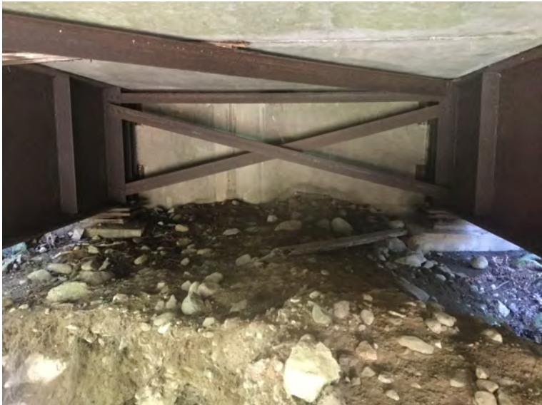
Left Bank Abutment when facing downstream
