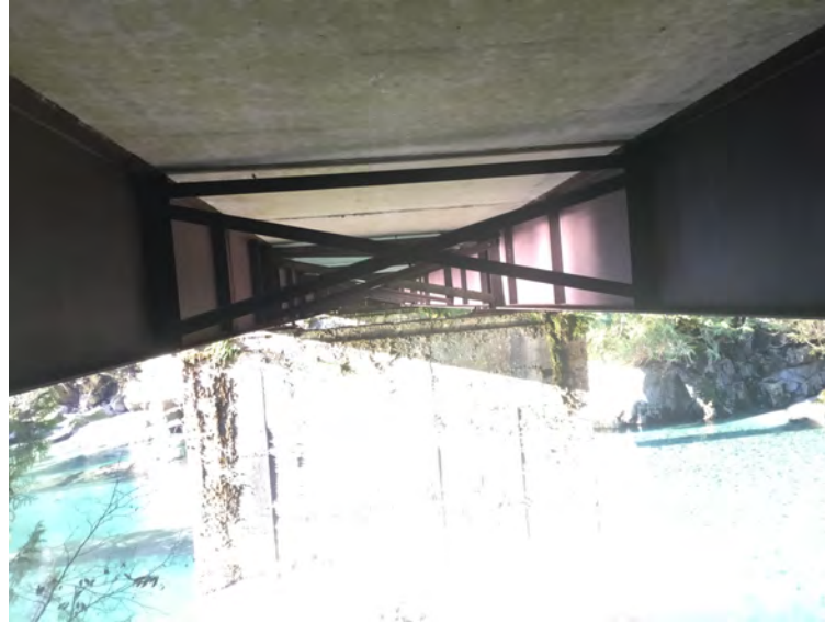
Left span superstructure
